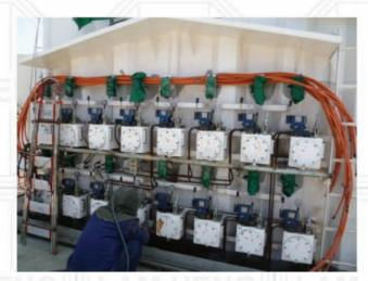
On-board installation and testing of hydraulic controlled system
