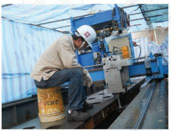
On-site Milling of 42m Cantilever Skidding **Beam**
