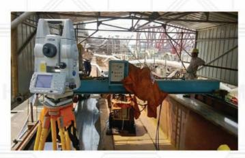
**Laser alignment using Total Station**
